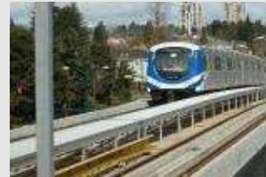
Rail signalling systems
